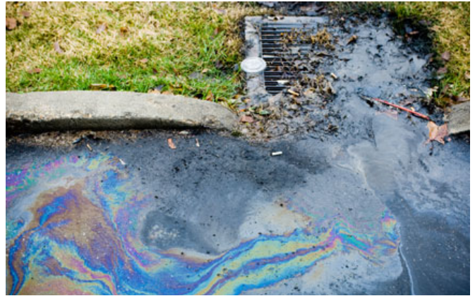
This discharge to a storm sewer delivers contaminants (motor oil, trash and organic debris) directly to a nearby stream.
