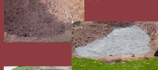
Step 2 - Layer of stone is added (above)
