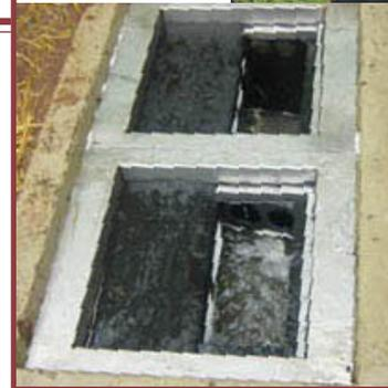
Inlet protection unit placed in stormwater inlet.
