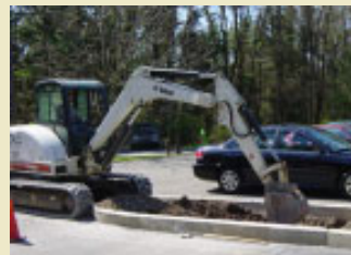
1. (above) Site is excavated.
