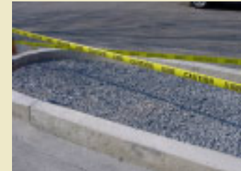
2. (above) Stone base layer is poured, spread and graded.
