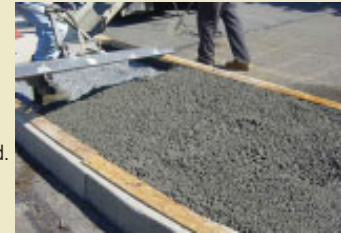
4. (above) Concrete is leveled with a screed.
