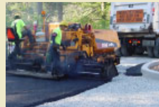
5. (above) Asphalt is laid.
