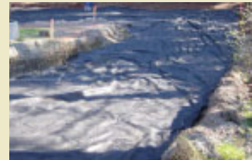
2. (above) Nonwoven geotextile material is laid over excavated area.
