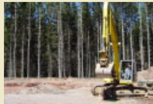
1. (above) Site is excavated.
