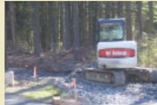
3. (above) Stone is spread and graded level.
