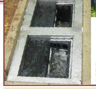
Inlet protection unit placed in stormwater inlet
