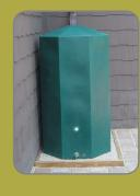
One of the most user-friendly BMPs from an installation standpoint, rain barrels can be implemented at any type of site and are a practical way for individual homeowners to practice water conservation. The barrel is connected to a downspout for capturing roof runoff. Runoff is stored in the barrel for later use. A garden
