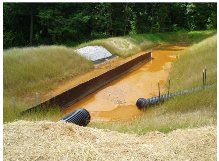
SEDIMENT TRAP - This sediment trap collects runoff from the disturbed site. Note the baffling to increase flow length. From Erosion and Sediment Pollution Control Program Manual, PADEP, March 2012 Courtesy of York County Conservation District
