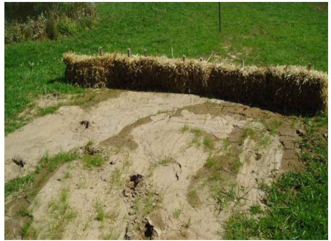
AN EXAMPLE OF STRAW BALES – Note the sediment accumulation upslope of the bales From Erosion and Sediment Pollution Control Program Manual, PADEP, March 2012 Courtesy of York County Conservation District
