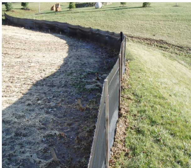
AN EXAMPLE OF FILTER FABRIC FENCE – This is a 30 inch reinforced fence.
