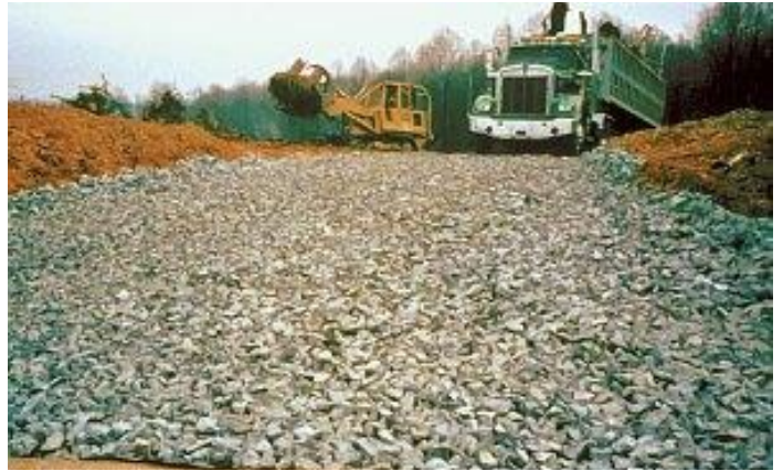
AN EXAMPLE OF ROCK CONSTRUCTION ENTRANCE - From Erosion and Sediment Pollution Control Program Manual, PADEP, March 2012 Courtesy Lake County Stormwater Management Department, Ohio
