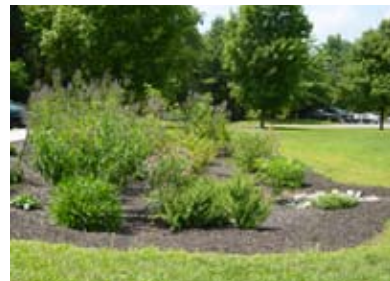
Rain Gardens filter pollutants and infiltrate runoff into the ground.
